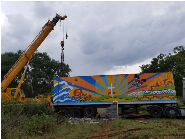
Container being offloaded by a crane
